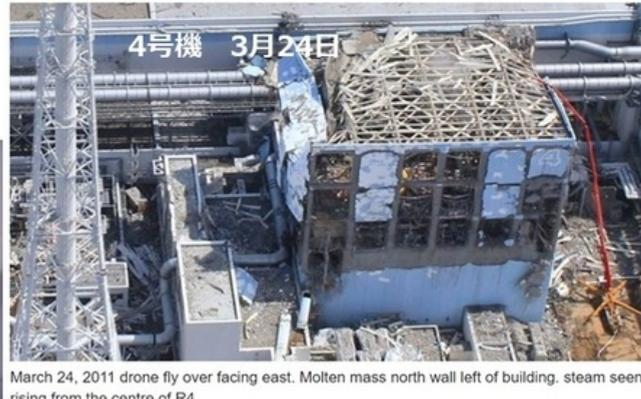
March 24, 2011 drone fly over facing east. Molten mass north wall left of building. steam seen rising from the centre of R4
