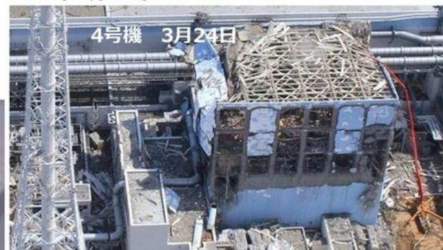
March 24, 2011 drone fly over facing east. Molten mass north wall left of building. steam seen rising from the centre of R4
