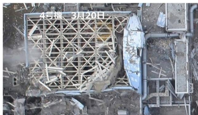
March 20, 2011 drone fly over looking straight down see the buckle in the north wall. SFP is still steaming away good thing that means there is water.
