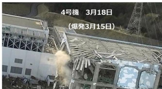
March 18, 2011 fly over. Yellow smoke seen rising up from R4SFP indicating fuel damage in the SFP!
